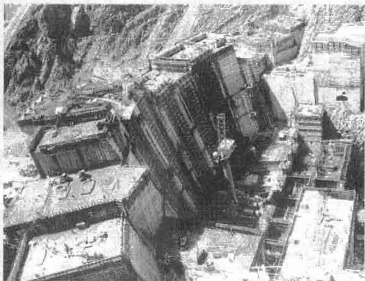
The Lijaxia Hydropower Station in construction.
