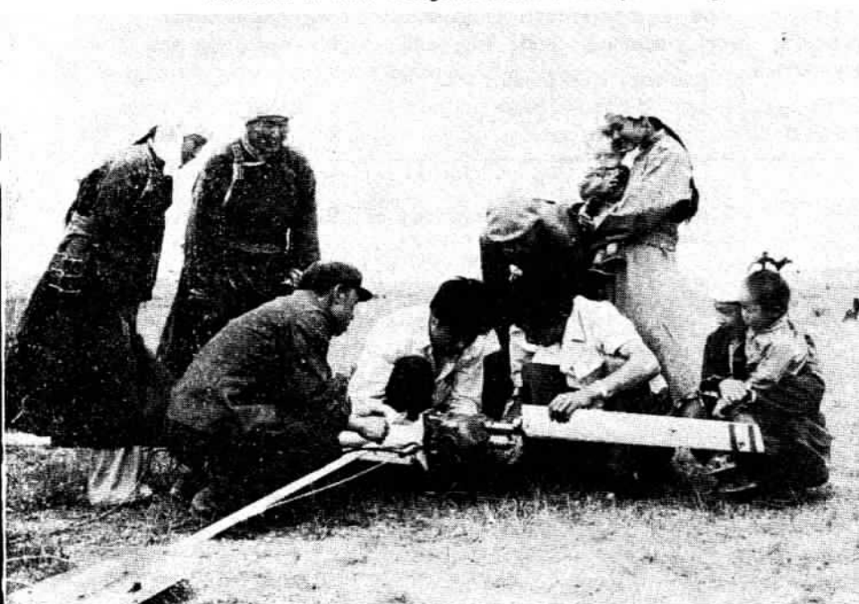
Herdsmen in Inner Mongolia install a wind-powered generator.
