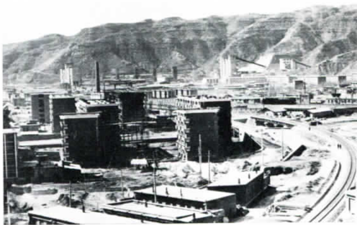
A view of the Gujiao Mining Area in Shanxi, the biggest coking base area to be completed during the Sixth Five-Year-Plan period.
