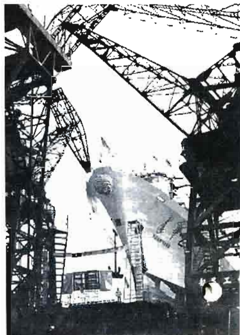
Building an ocean-going vessel for conducting surveys.
