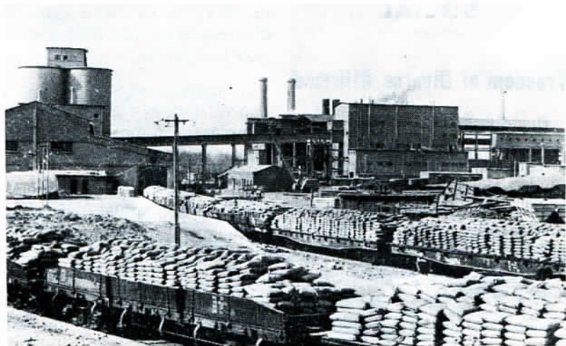
The newly built Xizhuozishan Cement Works in Inner Mongolia.
