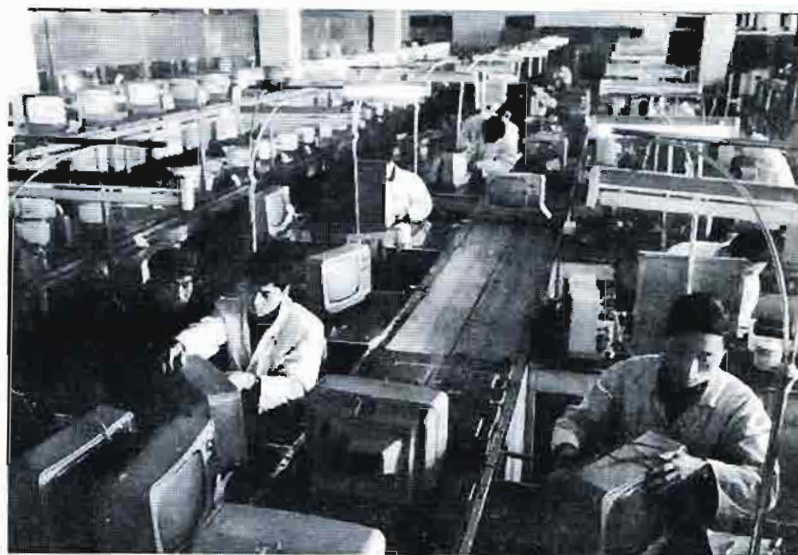
The general assembly line of the Tianjin Radio Factory where black-and-white TV sets are made.
