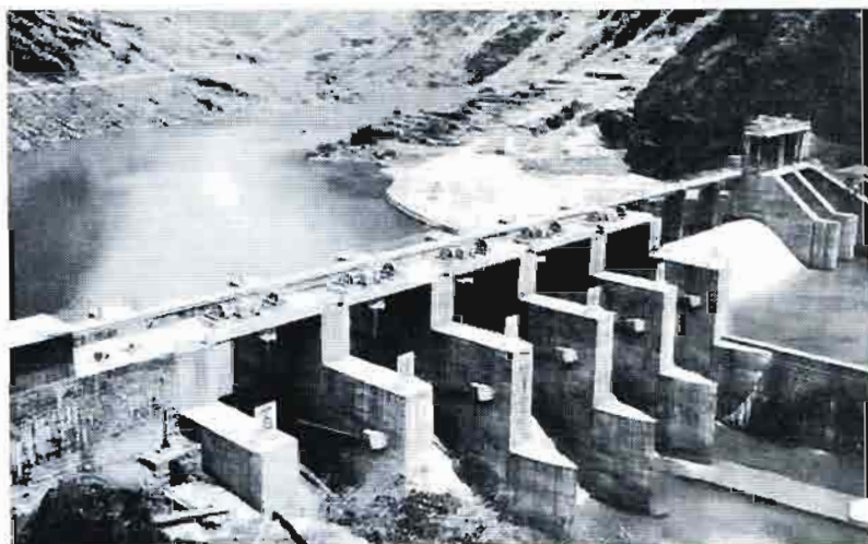
The Yuxi River water diversion project built and put in commission last year in Sichuan Province.
