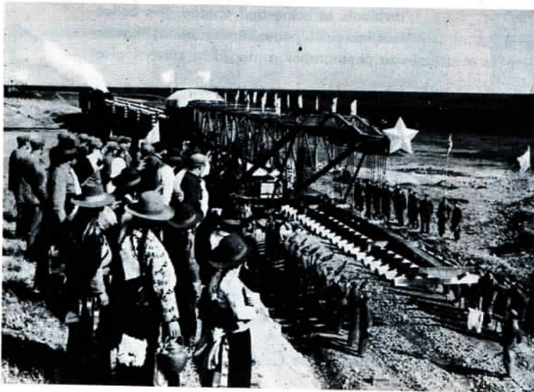
Qinghai-Tibet Railway under construction.
