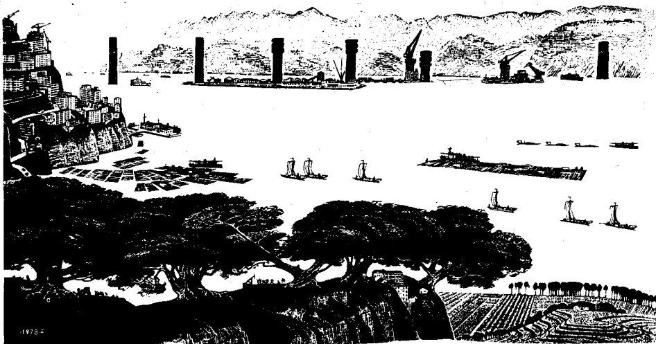
Building another bridge spanning the Changjiang River.
