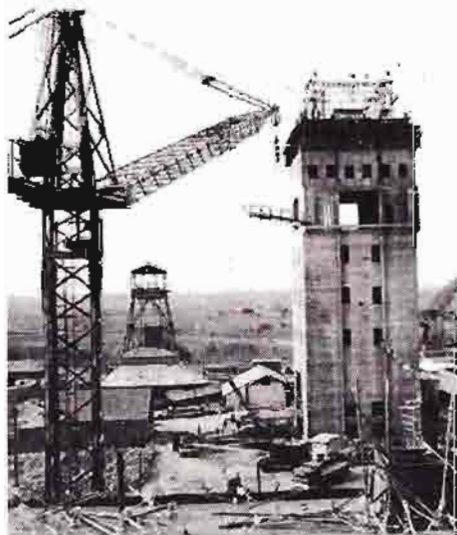
Yanzhou Colliery: Another big shaft under construction.
