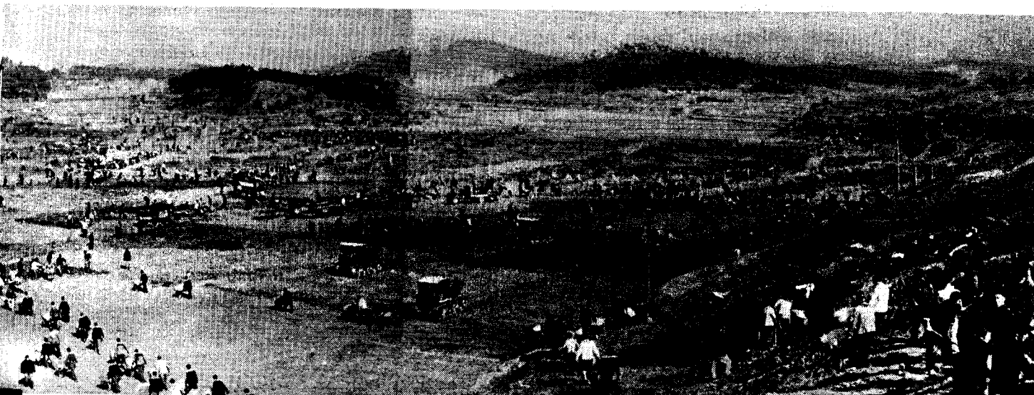
Reservoir under construction.
