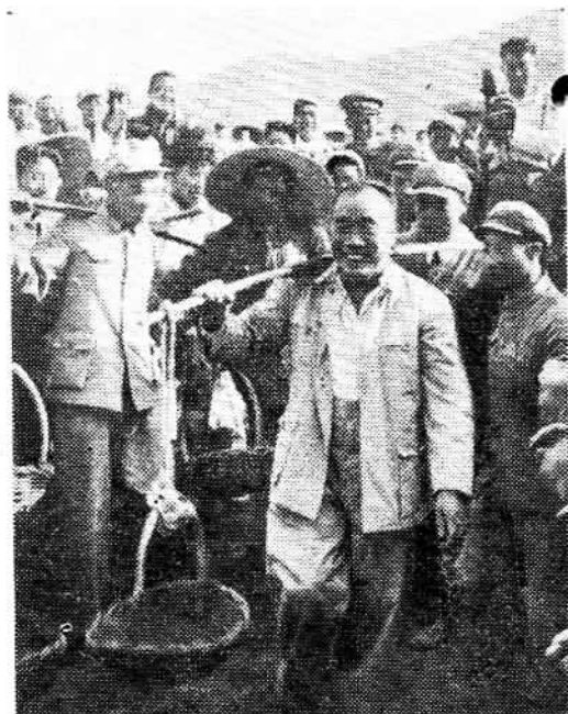
Comrade Chu Teh doing manual labour on the construction site of the Ming Tombs Reservoir on the outskirts of Peking in May 1953.
