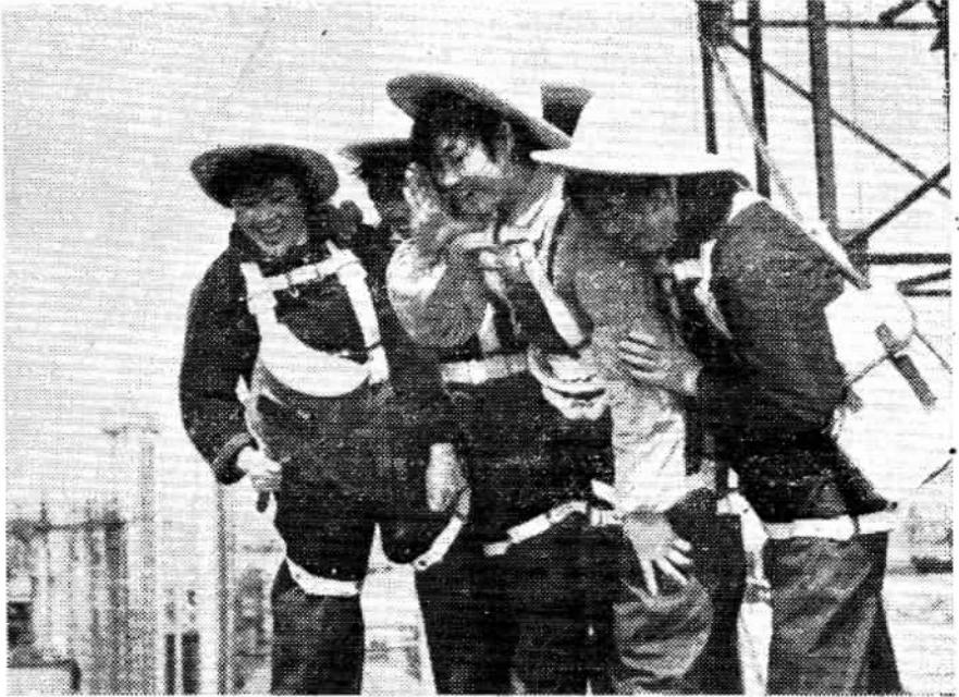
Women's crew working on a high scaffold.
