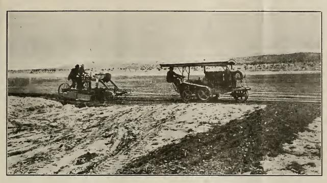
Leveling and scraping with caterpillar tractor.
