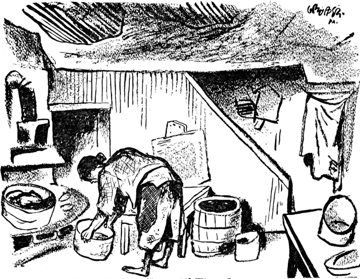
This is called a "home" by the Pittsburg Terminal Coal Co. - the place is in a cellar, rats running thru the houses, no water, and the stinking sewer at the door.
