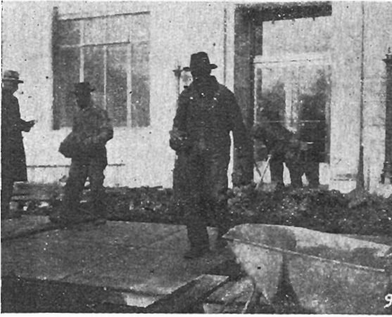
NEGRO WORKERS ON HOUSE WRECKING OPERATION
