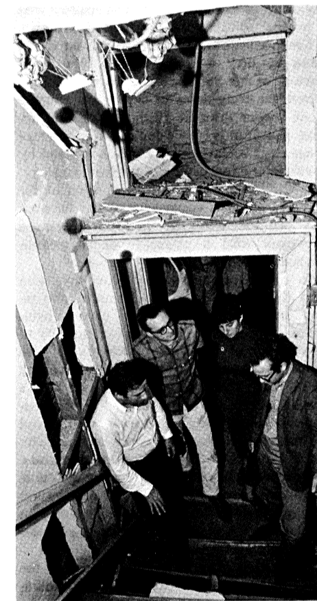
COMPLIMENTS OF CIA? Scene at entrance to L.A. SWP hall after bombing Oct. 16.
