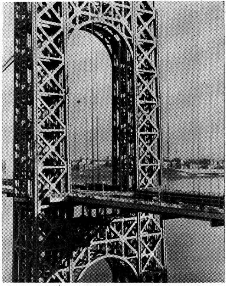
George Washington bridge. Patriotic New Yorkers consider it one of the world's most beautiful structures. To the Port Authority, the most beautiful feature seems to be the toll booth where motorists are stopped as if they were at the gates of a Middle Ages barony. Congressman Celler says tolls have paid for the bridge twice over.
