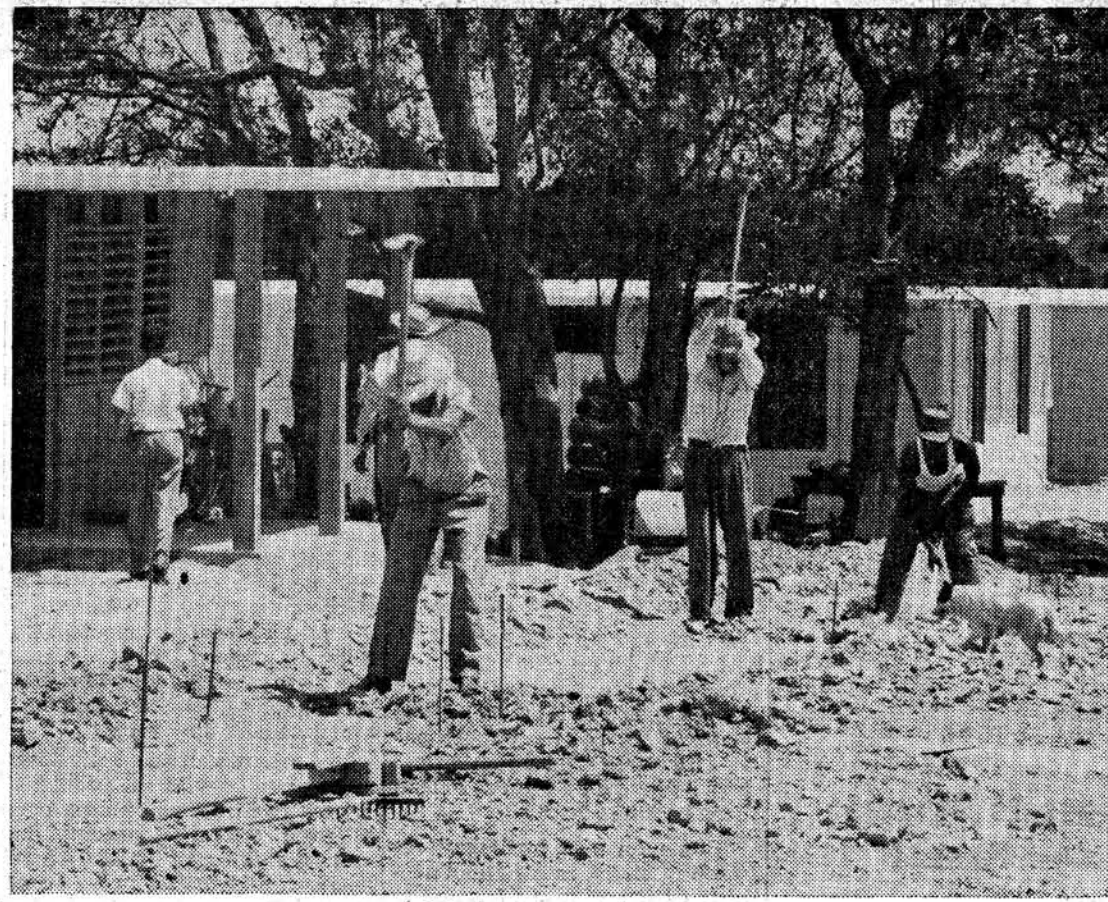
The old "bohio" with its palm-thatched roof and dirt floor is listed to go in Cuba. It will be replaced by model homes like these under construction — complete with inside plumbing. Members of the co-operatives don't mind the hard work or the primitive tools because they're building their own homes with government help. The perspective of a new Cuba, completely modernized, was made possible by the revolution that overthrew the Batista dictatorship.
