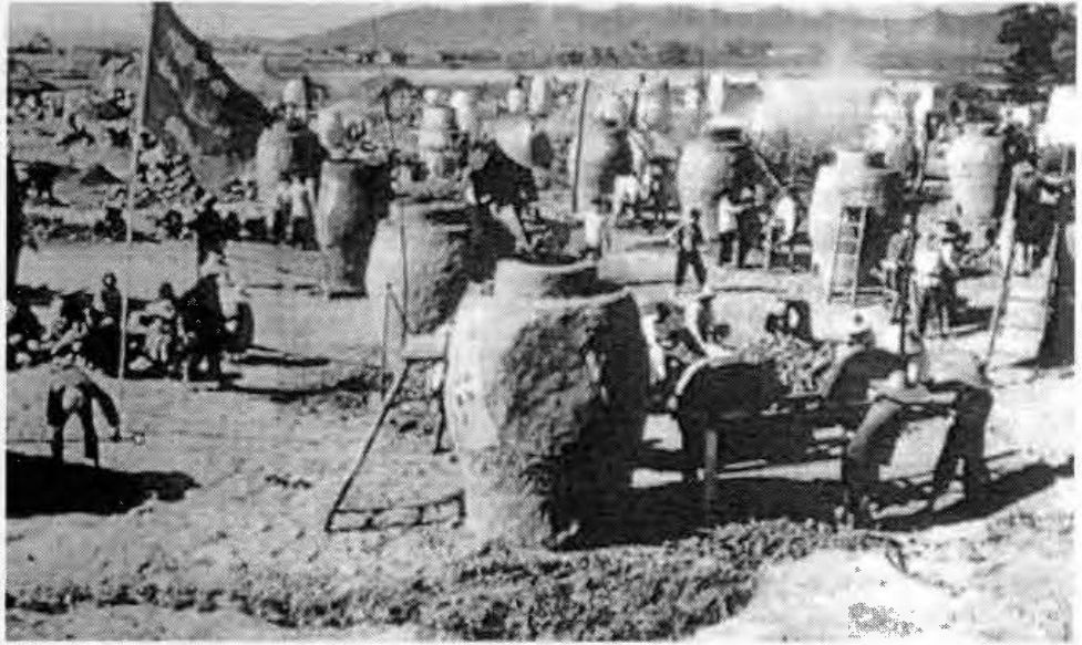
Primitive backyard furnaces during Mao's "Great Leap Forward" turned out to be disastrous, producing steel unfit for industrial use.
