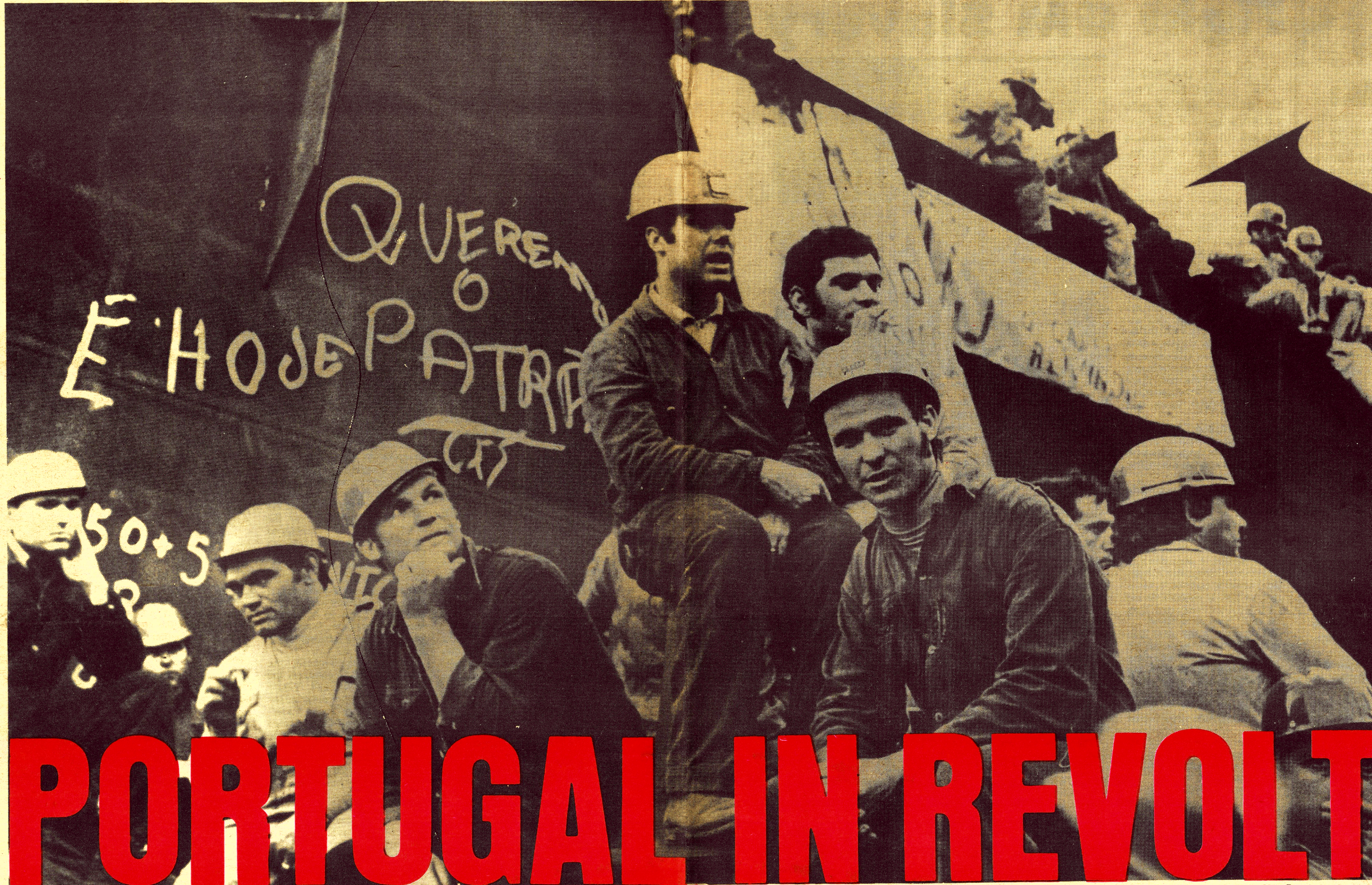
Workers at Lisnave shipyards during the occupation.
